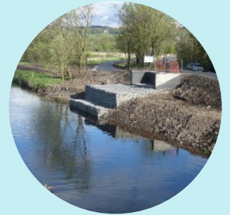
Foundations for the footbridge over the River Calder 2005
